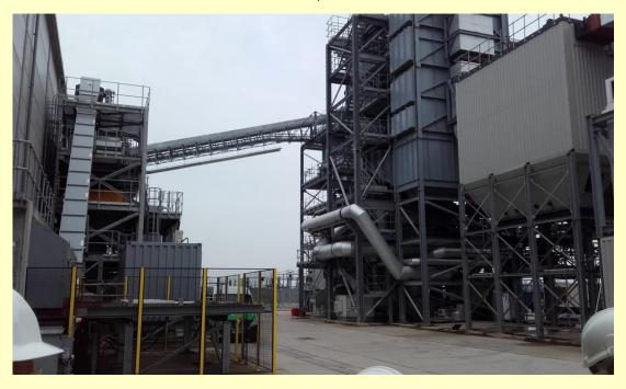
The operation of the site is, in essence, very simple. Waste wood arrives at the site, is burned to generate heat, which turns water into steam, which rotates a turbine, which creates electricity – which is then fed directly into the national grid. When fully operating, the site will generate enough electricity to power 40,000 homes!
